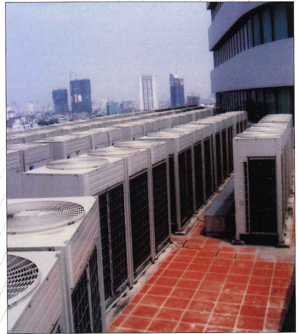
Viet Tower 189B Tây Sơn Install VRV Air Conditioning
